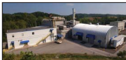
Transuranic Waste Processing Center
